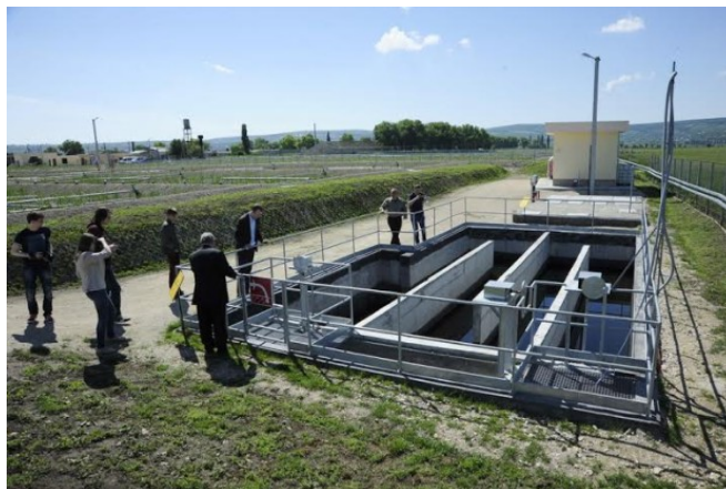
Figure 1. Reservoir from which the water treated at the Orhei treatment plant is discharged into the Raut river [3].
